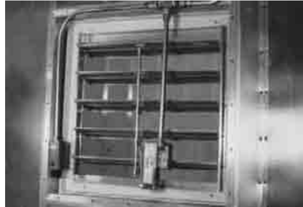
Figure 10. Moveable louvers.
